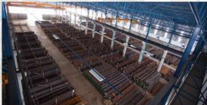
Special Steel Stockyard
